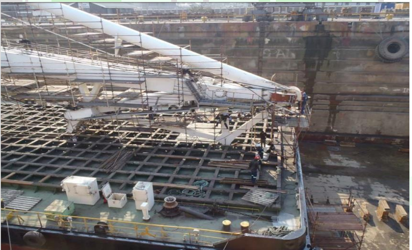
Transnet NPA 2014-Floating Crane Jib repair
